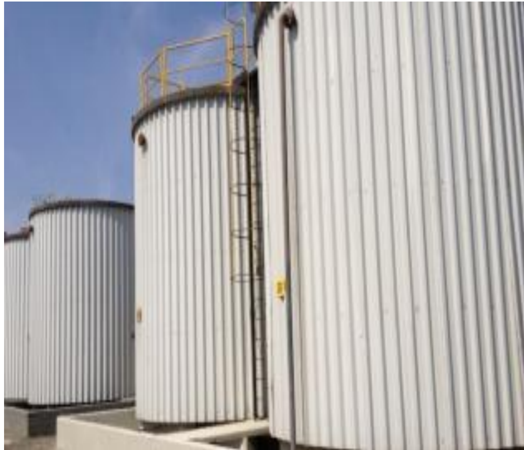
Silos containing original liquid Radwaste
